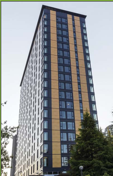
Brock Commons, UBC, Vancouver
